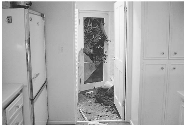
FIGURE 10.44 Two views of a debris flow. Upper photograph shows the area of detachment and the lower photograph shows how the flow forced its way into the house.
