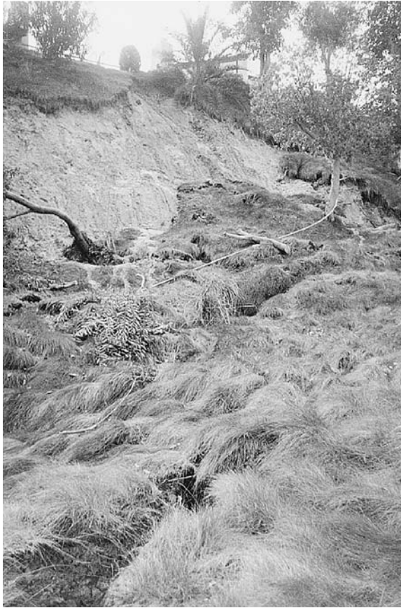
FIGURE 10.13 Surficial slope failure in a fill slope.
