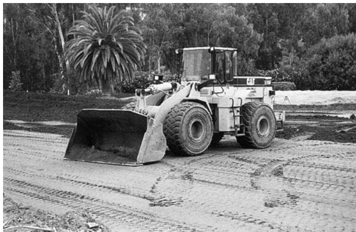
FIGURE 15.11 The loader can be used to move soil about the job site and compact the soil as structural fill.
