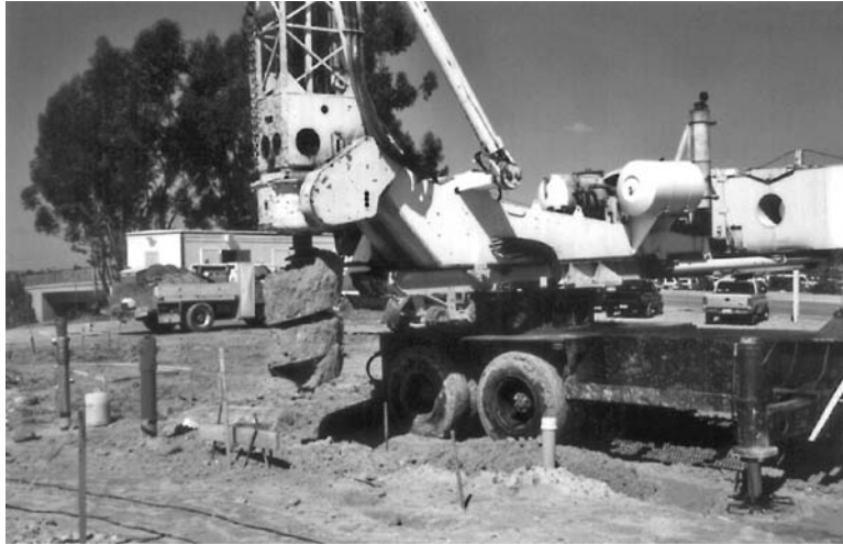
FIGURE 16.9 Truck-mounted auger drill rig used to excavate piers.
