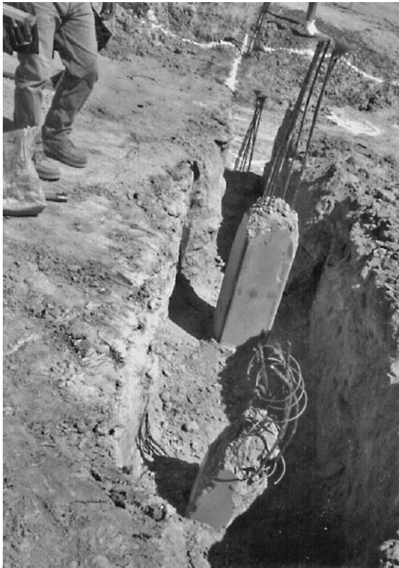
FIGURE 16.27 The prestressed concrete pile at the bottom of the picture is the same pile shown in Fig. 16.25. The pile near the center of the photograph is the replacement pile. The broken pile and the replacement pile will be attached to the grade beam.
