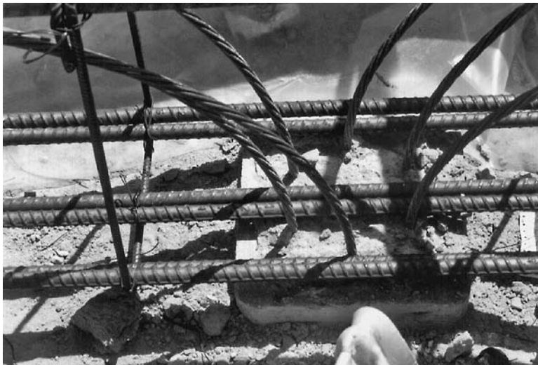
FIGURE 16.30 Close-up view of the top of a prestressed pile with the steel reinforcement from the grade beam positioned on top of the pile. The strands from the pile are attached to the steel reinforcement in the grade beam.
