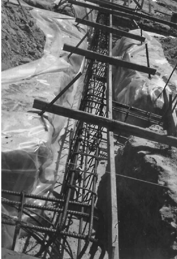
FIGURE 16.31 Overview of the steel reinforcement positioned within the grade beam excavation.
