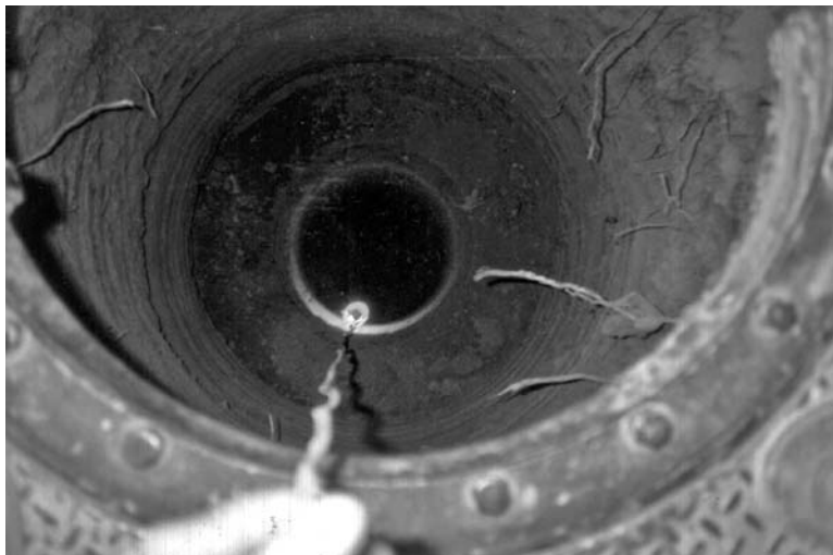
FIGURE 16.12 A light has been lowered to the bottom of the pier in order to observe embedment conditions.
