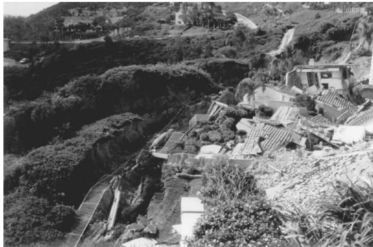
FIGURE 10.40 Laguna Niguel landslide: graben area created as the landslide moved downslope.
