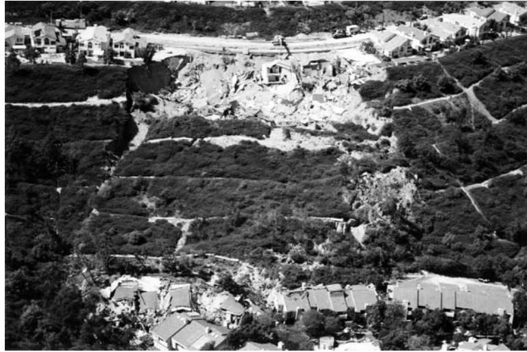
FIGURE 10.27 Overview of the Laguna Niguel landslide.
