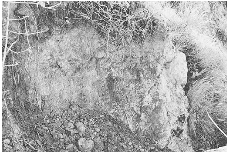
FIGURE 10.5 Location of rockfall.
