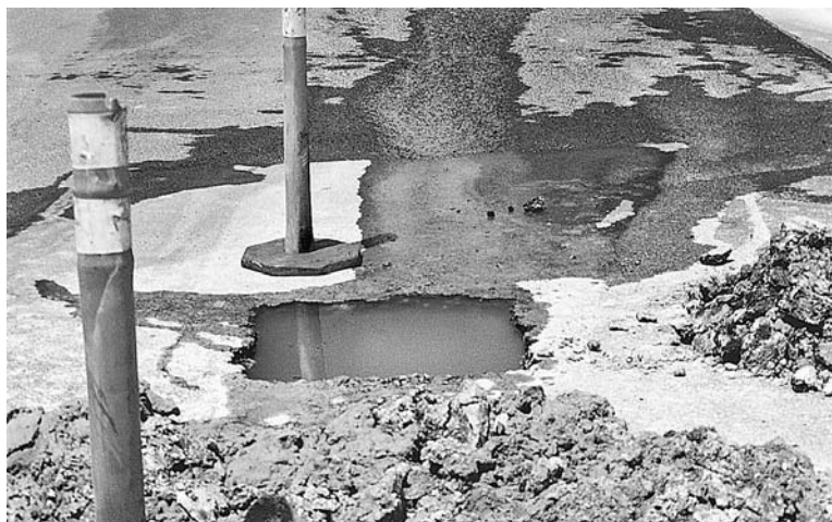
FIGURE 16.5 Groundwater exiting a test pit excavated into a pavement.
