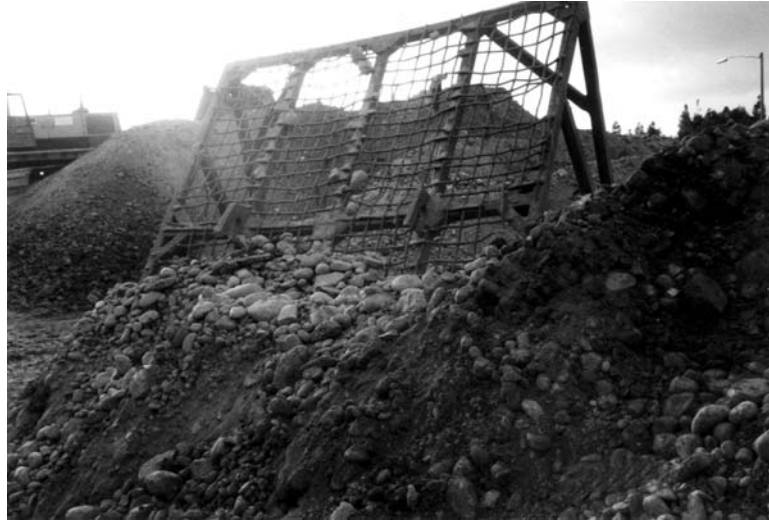
FIGURE 15.5 A screen has been set up in order to remove large-size rock fragments from the soil.
