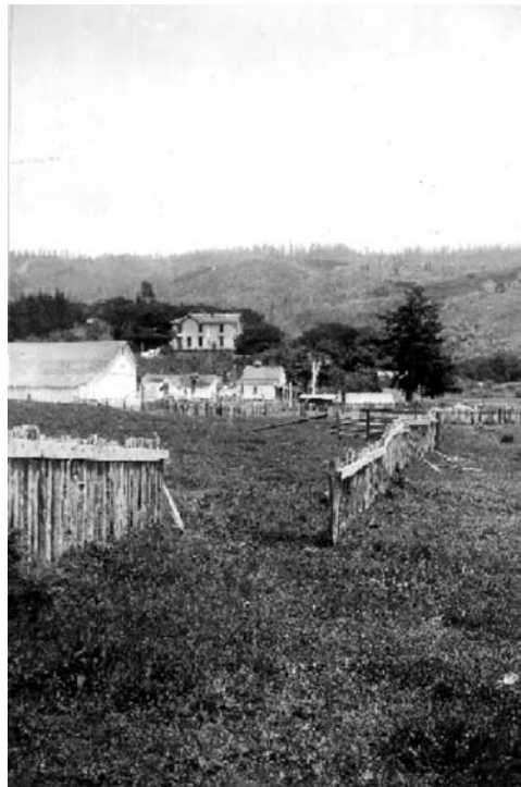
FIGURE 13.3 San Francisco earthquake, 1906. The fence has been offset 8.5 ft (2.6 m) by the San Andreas Fault displacement. The location is 0.5 mi (0.8 km) northwest of Woodville, Marin County, California. (Photograph courtesy of USGS).
