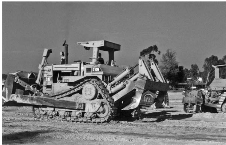
FIGURE 15.4 A Caterpillar D10 tractor/ripper that can be used to excavate rock.
