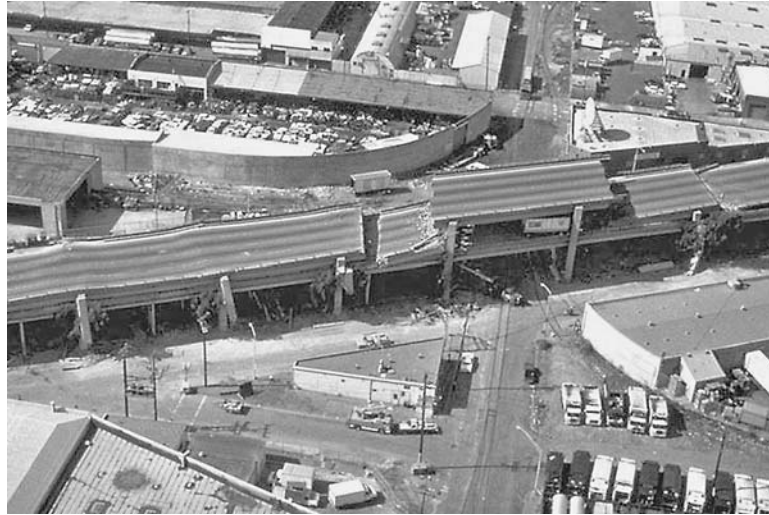
FIGURE 13.12 Overview of the collapse of the Cypress Street Viaduct caused by the Loma Prieta earthquake in California on October 17, 1989. (From USGS.)
