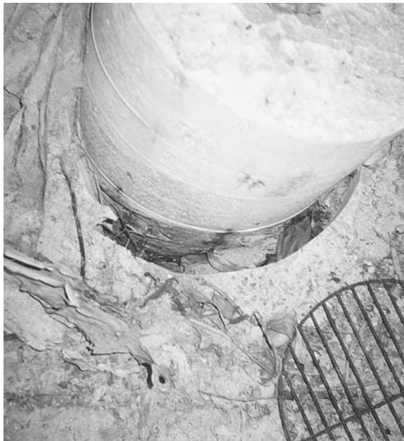
FIGURE 6.17 Soil movement around a concrete pier.
