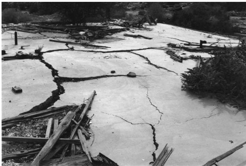
FIGURE 7.19 Foundation damage caused by ground fissures, Las Vegas, Nevada.
