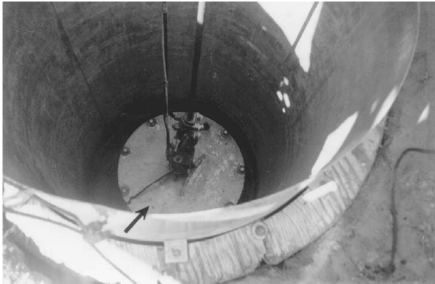
FIGURE 2.7 Downhole logging (arrow points to top of steel cage used for downhole logging).
