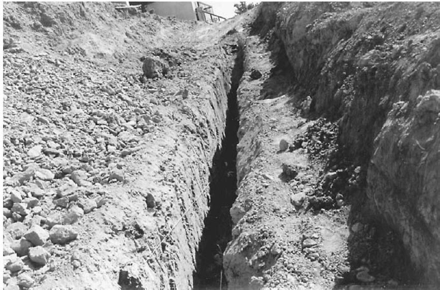
FIGURE 2.30 Backhoe trench for a fault study.
