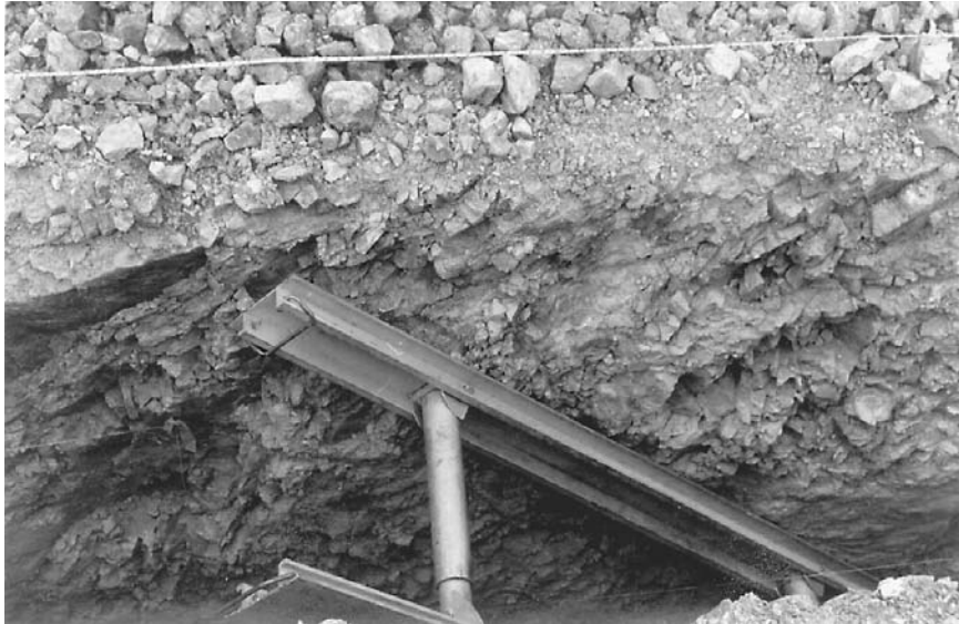
FIGURE 2.31 Close-up view of trench excavation.
