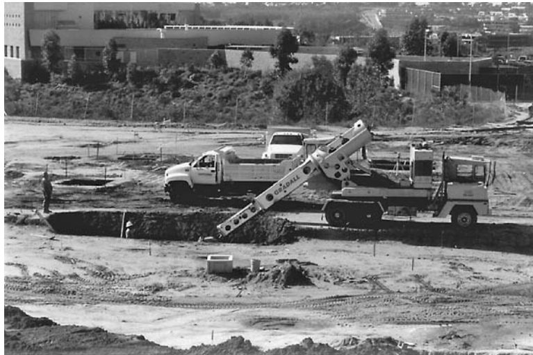
FIGURE 16.2 Excavation of footings.
