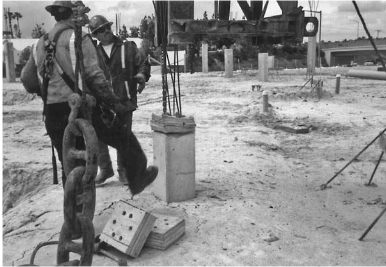
FIGURE 16.23 A prestressed concrete pile has been successfully driven to the bearing strata. The wood block shown on the top of the concrete pile was used as a cushion in order to protect the pile top from being crushed during the driving operation.
