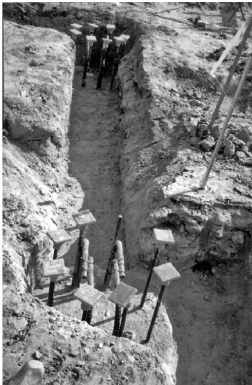
FIGURE 16.14 Excavation for the grade beam that will span between the two piers.
