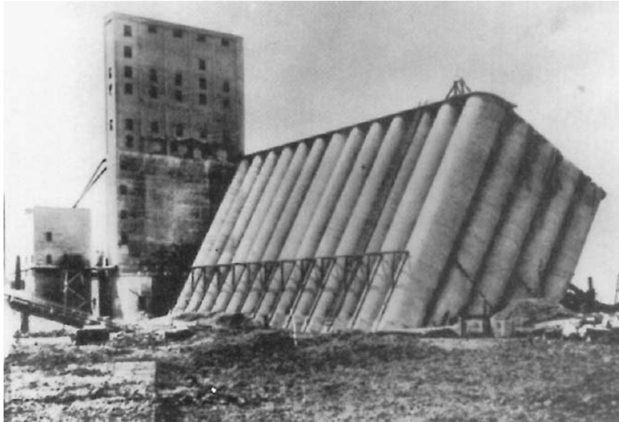
FIGURE 6.4 Transcona grain elevator failure.
