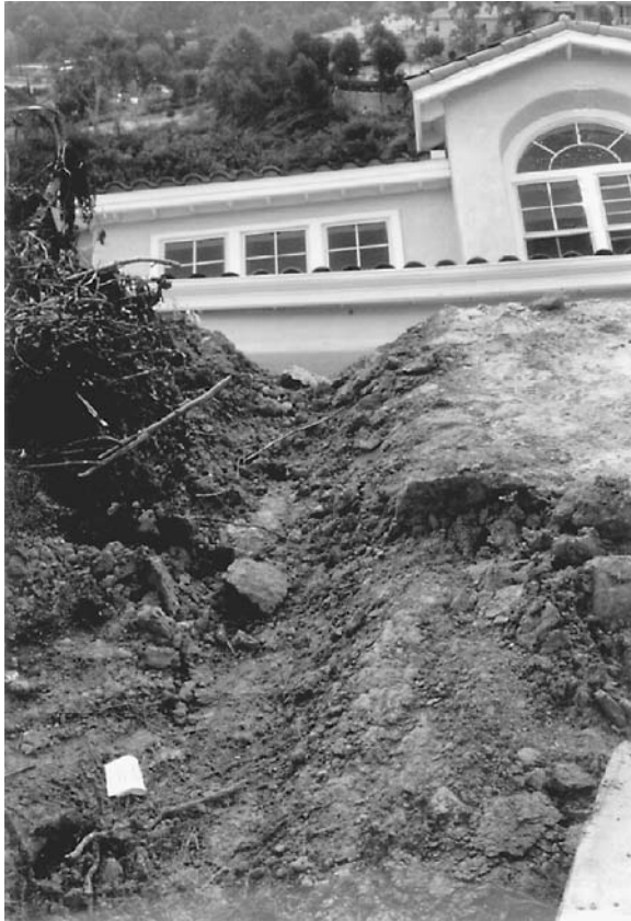
FIGURE 10.39 Laguna Niguel landslide: head of the landslide showing a house that has been pulled downslope.
