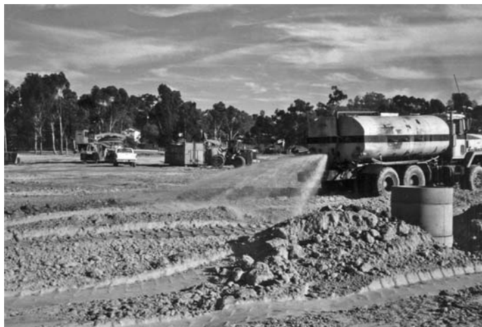
FIGURE 15.13 The water truck is adding water to fill that is in the process of being compacted.
