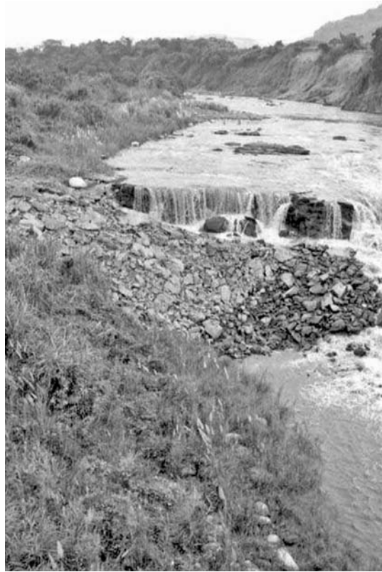
FIGURE 13.8 Close-up view of the waterfall shown in Fig. 13.7. The waterfall was created by the surface fault rupture associated with the Chi-chi (Taiwan) earthquake on September 21, 1999 and has an estimated height of 9 to 10 m. (Photograph from the USGS Earthquake Hazards Program, NEIC, Denver.)
