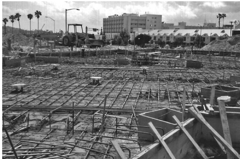
FIGURE 16.18 Positioning of the steel reinforcement for the floor slab.
