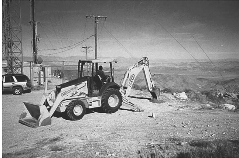
FIGURE 2.29 Backhoe in the process of excavating a test pit excavation.
