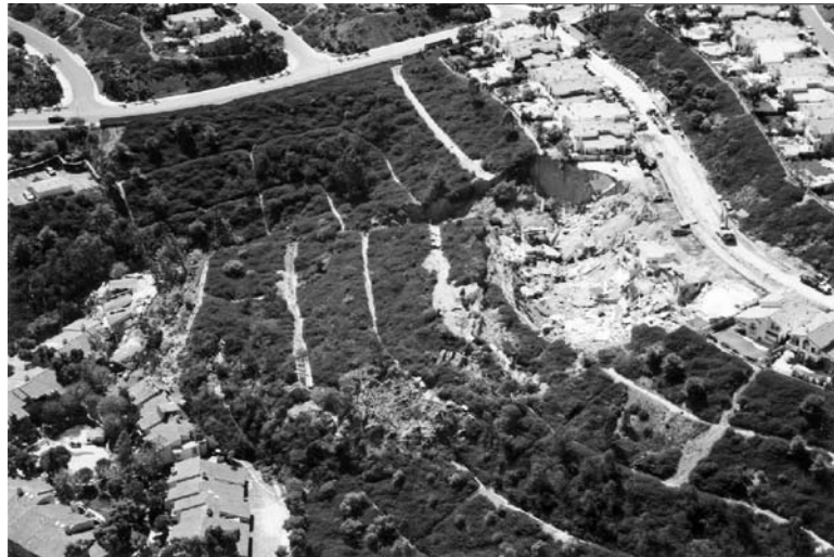
FIGURE 10.28 Overview of the Laguna Niguel landslide.
