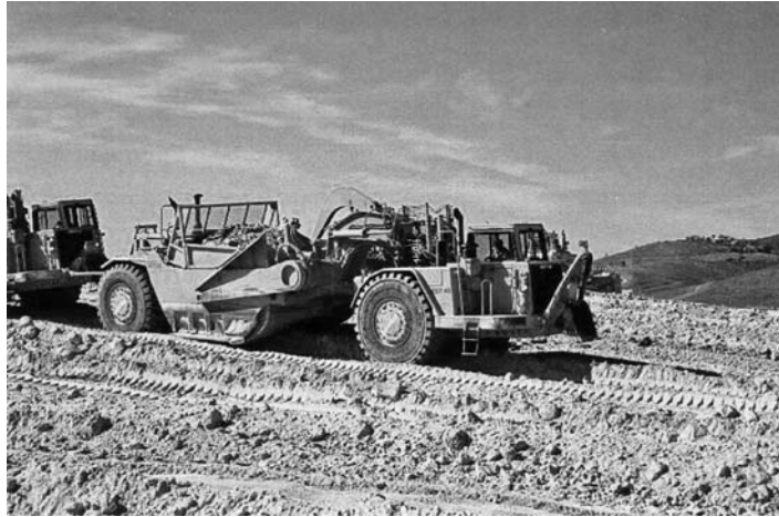
FIGURE 15.10 The scraper is used to excavate material from the borrow area, transport it to the site, dump it at the site, and then compact the soil.
