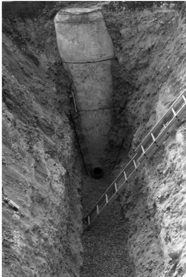
FIGURE 15.7 Utility trench excavation for a storm-drain line.
