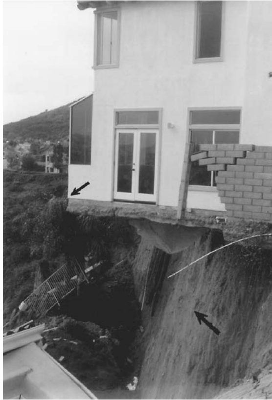
FIGURE 10.35 Laguna Niguel landslide: head of the landslide. (Note: The smaller arrow points to the corner of a house that is suspended in mid-air and the larger arrow points to the main scarp.)
