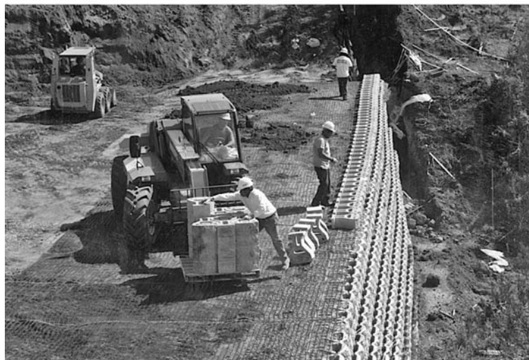
FIGURE 11.10 Two views of the installation of the geogrid for a mechanically stabilized earth retaining wall. The large arrows indicate the width of the mechanically stabilized zone and the small arrow points to a geogrid splice.
