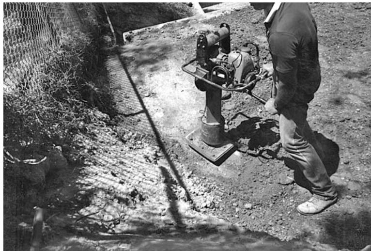
FIGURE 15.14 Hand-operated vibratory plate compactor used for compacting fill in tight spaces.
