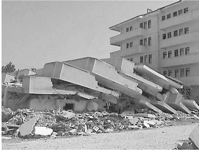
FIGURE 14.6 Pancaking of a building during the Kocaeli earthquake in Turkey on August 17, 1999. (Photograph by Mehmet Celebi, USGS.)
