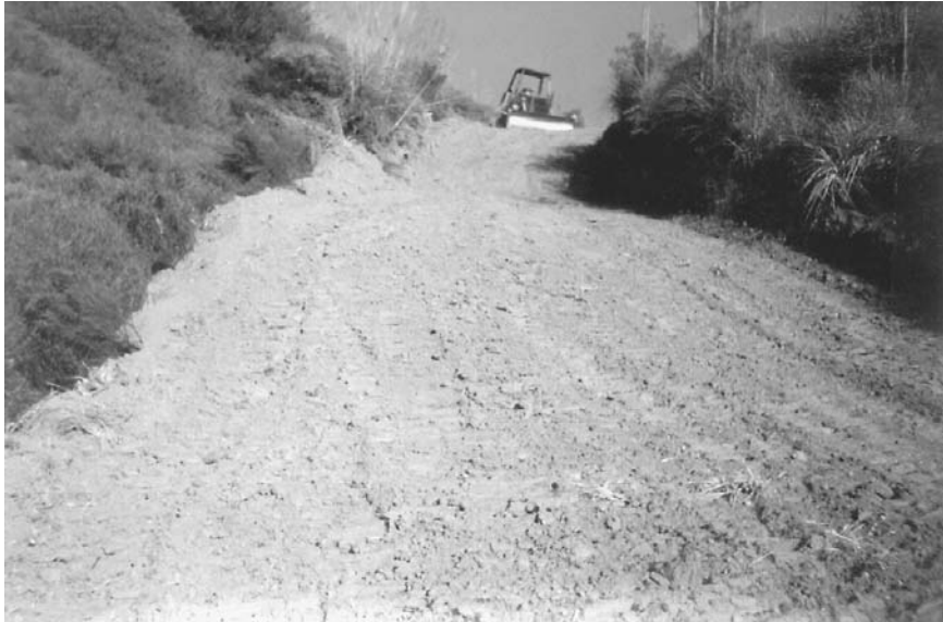
FIGURE 2.27 Construction of an access road for drilling equipment.
