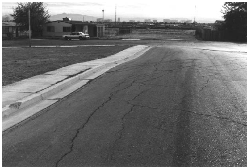
FIGURE 7.21 Settlement of the street and sidewalk due to ground fissures, Las Vegas, Nevada. Note that the Las Vegas strip is visible in the background of this photograph.
