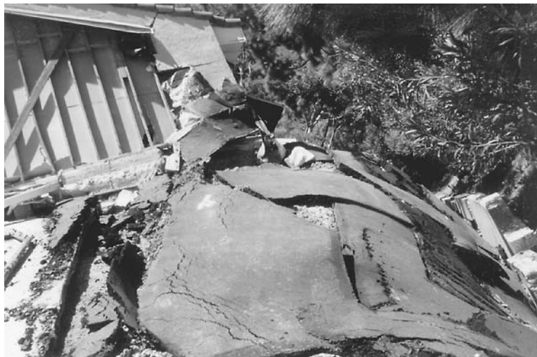
FIGURE 10.32 Laguna Niguel landslide: another view of the toe of the landslide where the road has been uplifted 20 ft.
