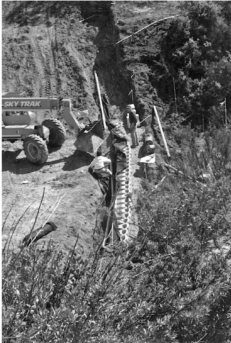
FIGURE 11.9 Excavation of key and installation of drainage system for a mechanically stabilized earth retaining wall.
