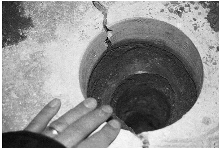
FIGURE 12.12 Excessive shrinkage crack in a concrete slab-on-grade foundation. The concrete has been cored and the crack is observed to penetrate the entire thickness of the concrete. Note that a visqueen moisture barrier is visible at the location of the core.
