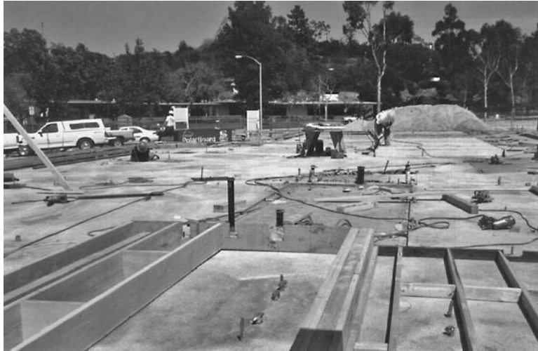
FIGURE 16.19 Concrete for the floor slab has been placed.
