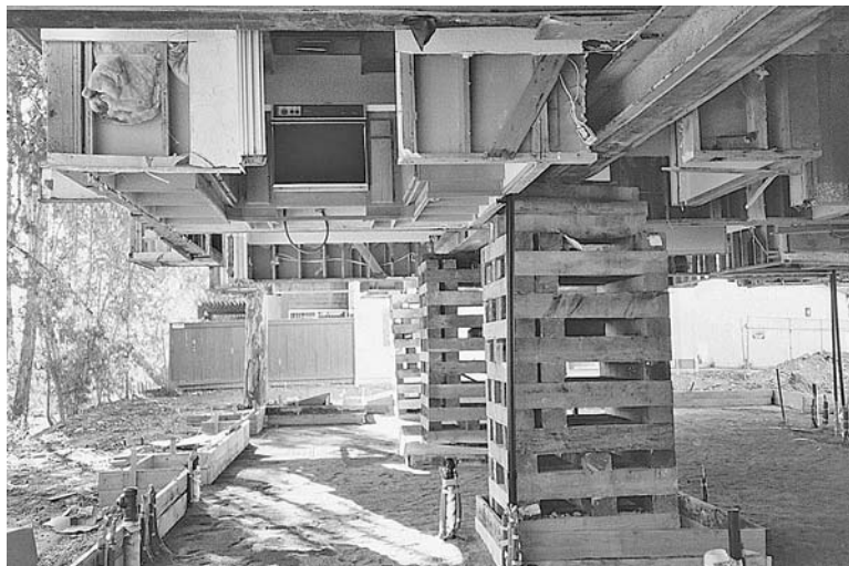
FIGURE 16.40 Construction of the mat foundation.
