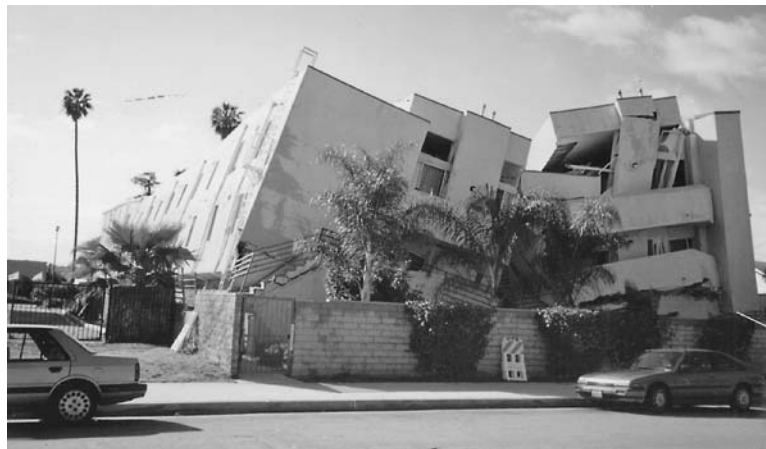
FIGURE 14.2 Building collapse caused by a soft story due to the parking garage on the first floor. The building collapse occurred during the Northridge earthquake in California on January 17, 1994.
